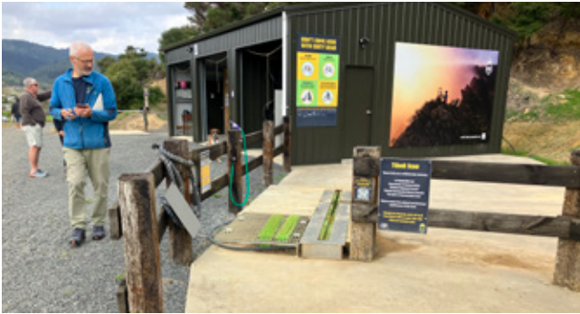
The wash station is designed for bikes and helps stop the spread of Kauri dieback disease
